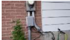
Pic. 2: Main power conduit appears split
