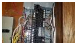
Pic. 26: 100 amp breaker panel with aluminum (70%) and copper (30%) wire
