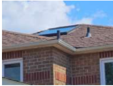
Pic. 2: Roof covering
