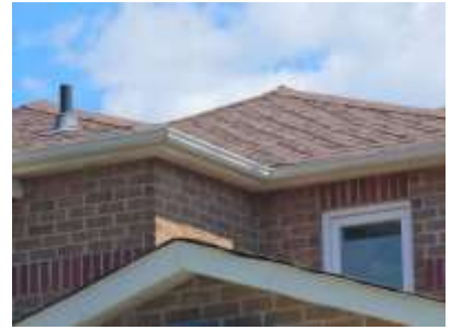
Pic. 3: Roof covering
