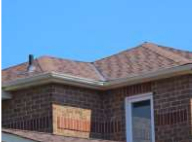
Pic. 4: Roof covering
