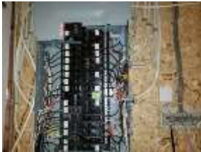
Pic. 33: 100 amp breaker panel
