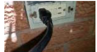
Pic. 4: Rear GFCI outlet defective
