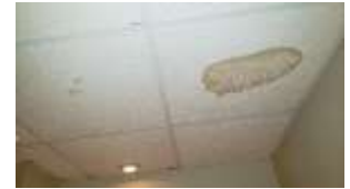
Pic. 202: Old water marks on ceiling tiles in basement bath
