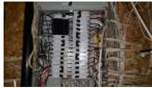
Pic. 235: 100 amp breaker panel with all copper wire
