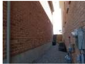
Pic. 7: Side view
