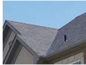
Pic. 3: Roof covering
