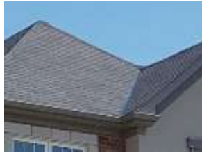
Pic. 2: Roof covering
