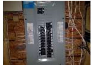
Pic. 32: 100 amp breaker panel with all copper wire
