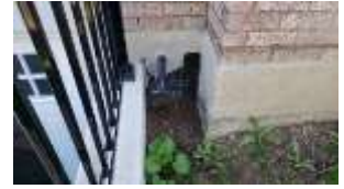
Pic. 4: Sump pump drain line – recommend extending away from foundation
