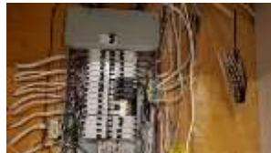
Pic. 46: Main electrical panel 100 amp service
