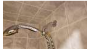
Pic. 39: Basement bath shower head leaking at threads
