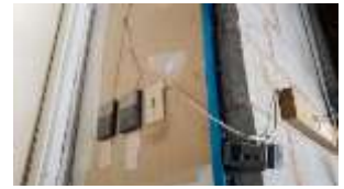
Pic. 12: Homeowner / handyman wiring for light in garage
