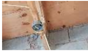
Pic. 11: Junction box in garage needs a cover plate
