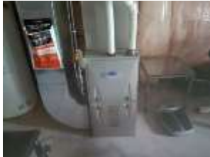
Image 29: Updated high efficiency gas furnace
