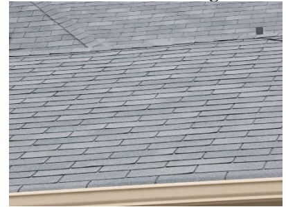
Pic. 6: Rear roof covering
