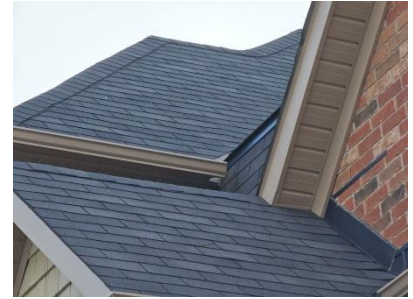
Pic. 3: Front roof covering
