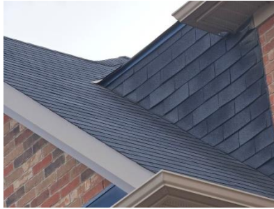
Pic. 2: Front roof covering
