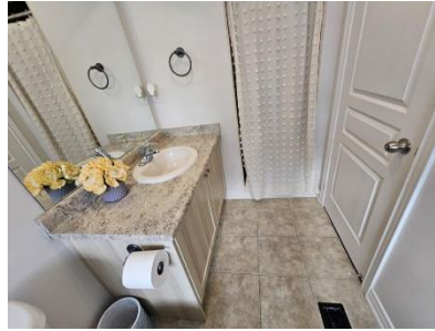
Pic. 17: Primary bathroom
