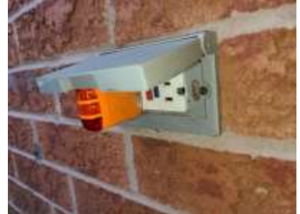
Pic. 6: Rear GFCI outlet needs replacement
