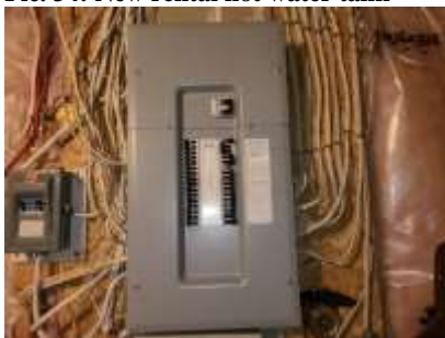
Pic. 37: 100 amp breaker panel with all copper wire
