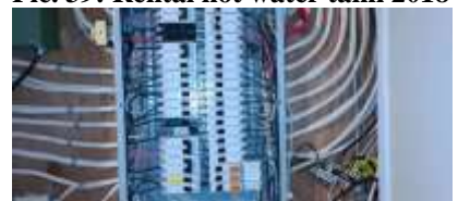
Pic. 42: 200 amp main breaker panel
