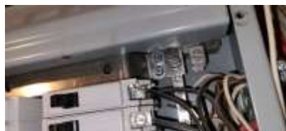
Pic. 44: Double tapped breaker
