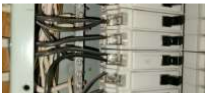
Pic. 43: Double tapped breakers
