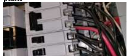
Pic. 45: Double tapped breakers
