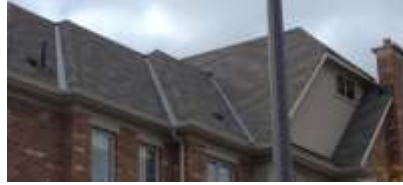
Pic. 2: Original roof covering
