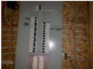
Pic. 33: 100 amp breaker panel
