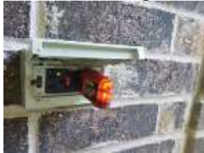
Pic. 6: Rear GFCI defective – needs replacement
