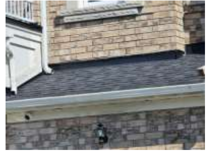
Pic. 3: Updated roof covering
