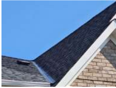
Pic. 2: Updated roof covering
