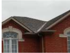
Pic. 2: Roof covering
