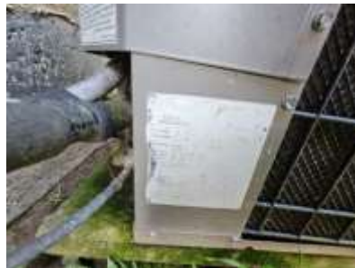
Pic. 8: AC data plate faded; age could not be determined
