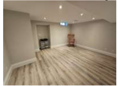
Pic. 30: Basement room
