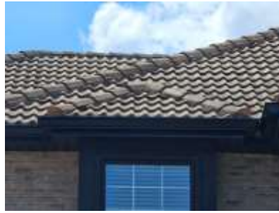
Pic. 2: Roof covering
