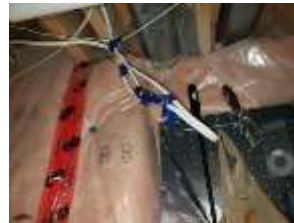
Pic. 35: Open air wiring junction needs to be placed in proper junction box
