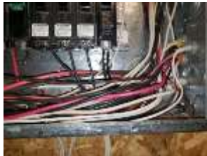
Pic. 34: Double tapped breaker
