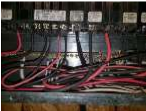
Pic. 33: Double tapped breaker
