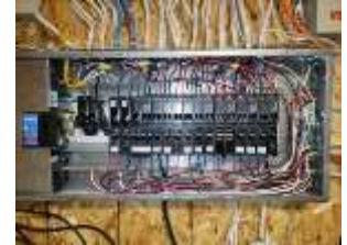
Pic. 32: 200 amp breaker panel
