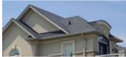
Pic. 2: Roof covering
