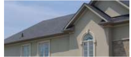
Pic. 3: Roof covering
