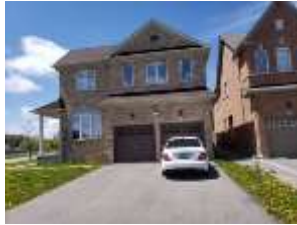
Pic. 2: Garage view
