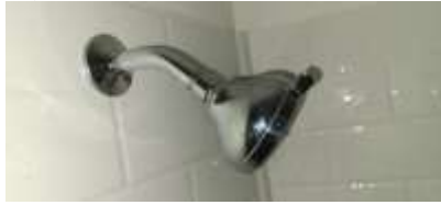
Pic. 23: Shower head leaks – plumbers tape recommended for the threads
