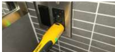
Pic. 17: GFCI outlet in main floor bath won't trip – replace accordingly
