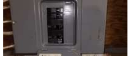
Pic. 27: Pony panel – Opening in the front of the panel needs to be sealed
