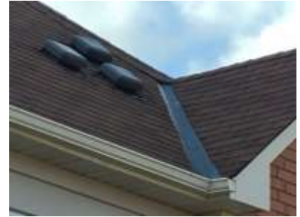
Pic. 3: Original roof covering
