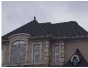
Pic. 2: Roof covering
