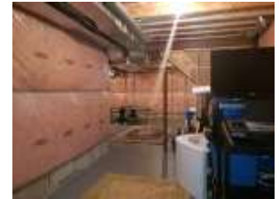
Pic. 36: Unfinished lower basement
