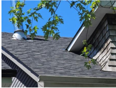
Pic. 2: Updated roof covering
