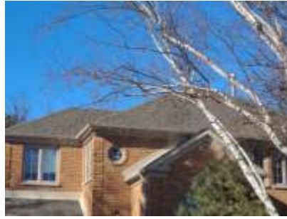
Pic. 2: Updated roof covering
