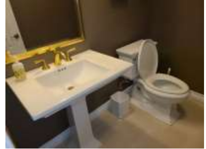
Pic. 36: Basement bath
