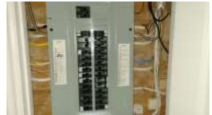
Pic. 27: 100 amp breaker panel
