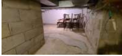
Pic. 26: Crawl space
