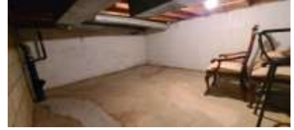
Pic. 27: Crawl space
