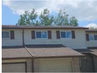
Pic. 2: Updated roof covering
