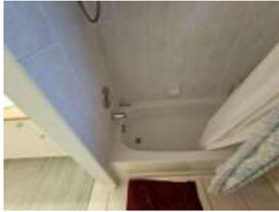
Pic. 17: 2 nd floor bath
