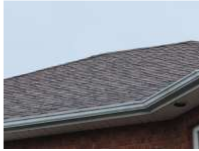
Pic. 2: Roof covering
