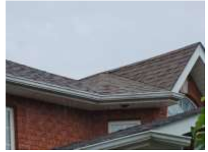
Pic. 3: Roof covering
