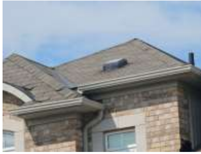
Pic. 2: Roof covering
