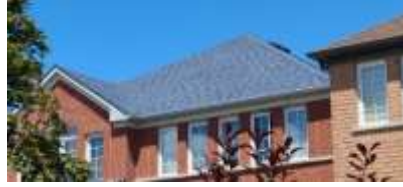
Pic. 2: Updated roof covering
