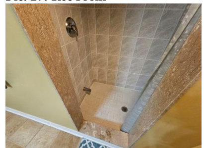
Pic. 30: Basement bathroom
