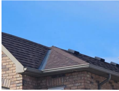
Pic. 2: Updated roof covering
