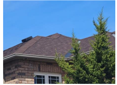
Pic. 3: Updated roof covering
