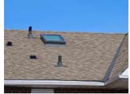
Pic. 3: Updated roof covering
