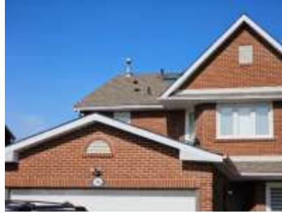
Pic. 2: Updated roof covering
