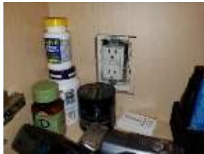
Pic. 14: Outlet loose and cover plate missing
