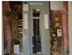
Pic. 43: 200 amp breaker panel
