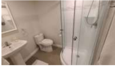
Pic. 29: Basement bath
