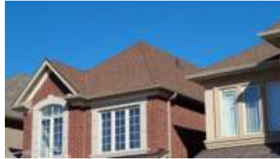
Pic. 2: Original roof covering
