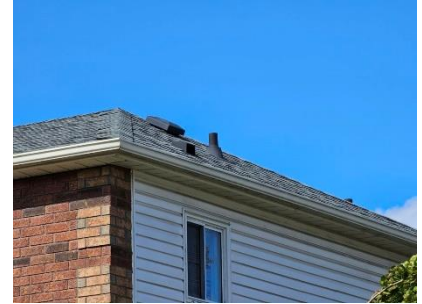
Pic. 3: Updated roof covering
