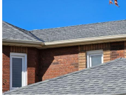
Pic. 2: Updated roof covering
