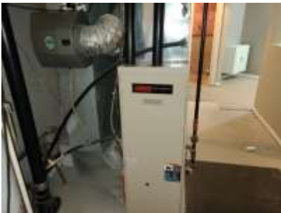
Pic. 22: Original gas furnace to be replaced before closing
