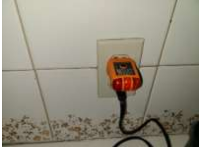
Pic. 19: Reverse polarity outlet in kitchen
