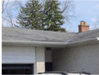
Pic. 2: Roof covering – aging but still functional
