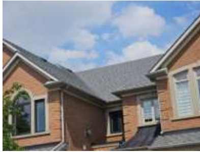
Pic. 2: Updated roof covering
