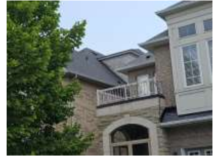
Pic. 3: Updated roof covering
