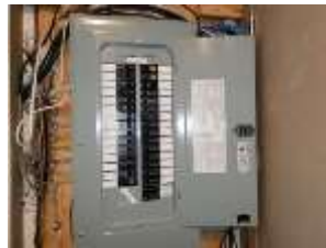
Pic. 6: 100 amp breaker panel
