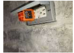
Pic. 4: Exterior GFCI needs to be replaced
