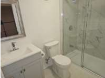
Pic. 34: Basement bathroom
