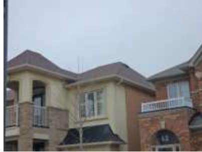
Pic. 2: Original roof covering
