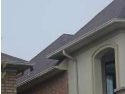
Pic. 4: Original roof covering
