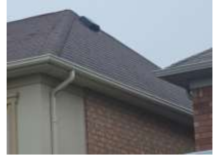
Pic. 3: Original roof covering
