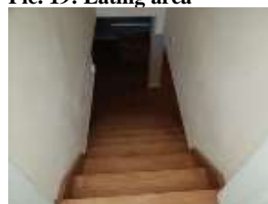
Pic. 23: Handrailing needed for basement stairwell
