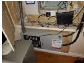
Pic. 34: Generator sub panel
