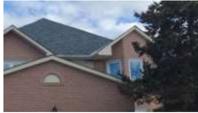
Pic. 2: Updated roof covering
