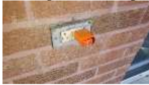
Pic. 6: Rear GFCI needs replacement
