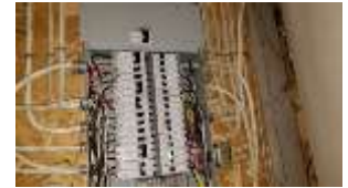
Pic. 40: 100 amp breaker panel
