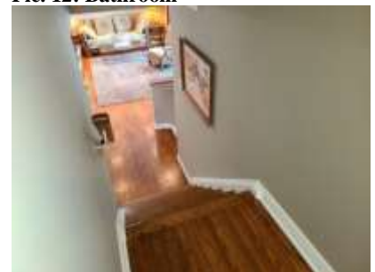
Pic. 15: Handrailing advised for stairwell
