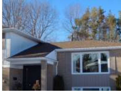
Pic. 2: Updated roof covering
