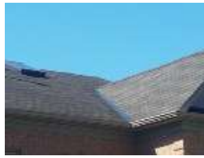
Pic. 2: Roof covering
