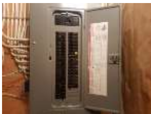
Pic. 37: 200 amp breaker panel with all copper wire
