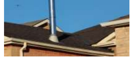
Pic. 3: Roof covering
