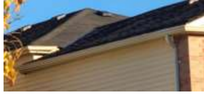
Pic. 2: Roof covering
