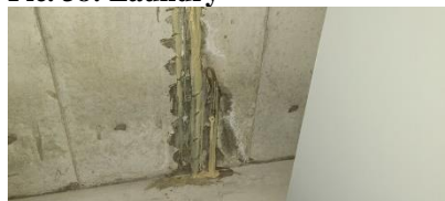
Pic. 41: Foundation repair #2
