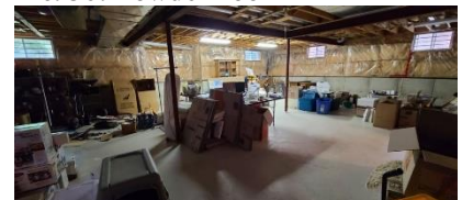
Pic. 39: Unfinished basement
