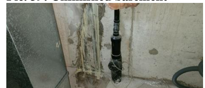
Pic. 42: Foundation repair #3
