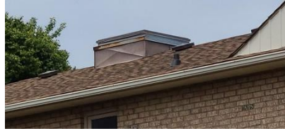
Pic. 2: Updated roof covering
