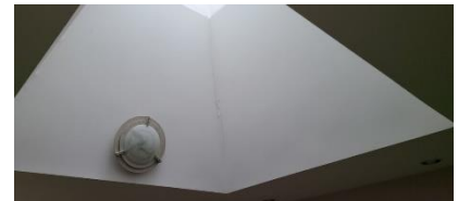
Pic. 27: Main skylight
