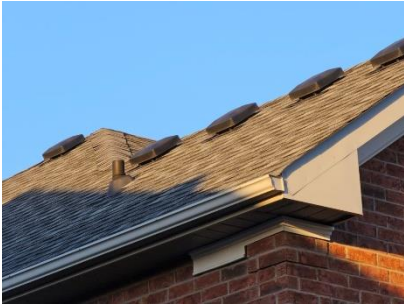
Pic. 4: Updated roof covering
