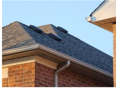
Pic. 2: Updated roof covering
