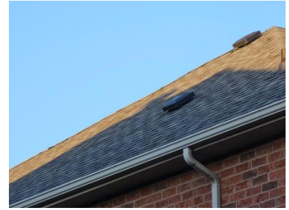
Pic. 3: Updated roof covering
