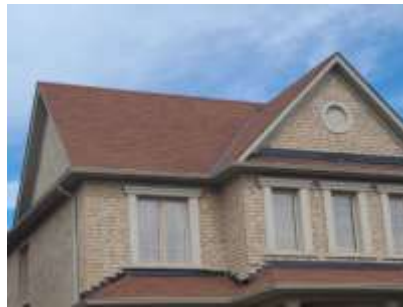
Pic. 2: Roof covering
