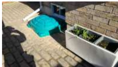
Pic. 8: Rear patio sloped towards the foundation recommend regrading
