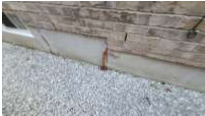
Pic. 4: Repaired foundation cracks
