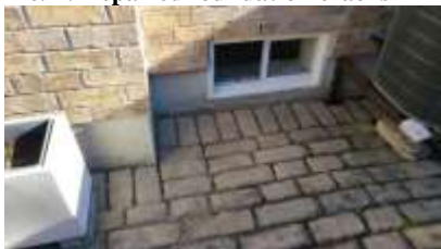
Pic. 7: Rear patio sloped towards the foundation recommend regrading
