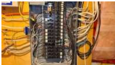
Pic. 32: 100 amp breaker panel with all copper wire
